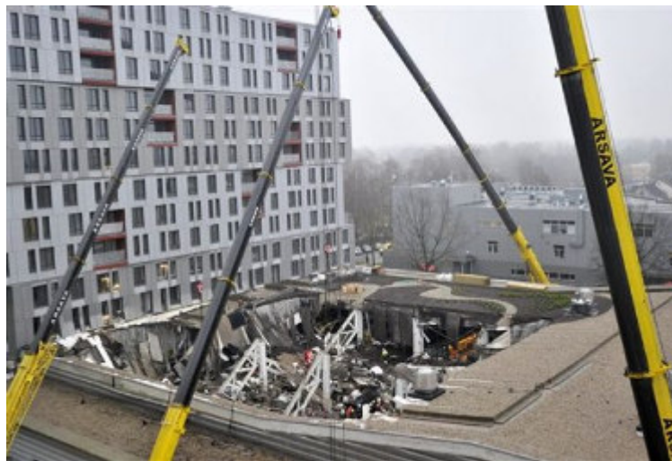
Fig. 1. Progressive collapse in Riga supermarket Maxima
