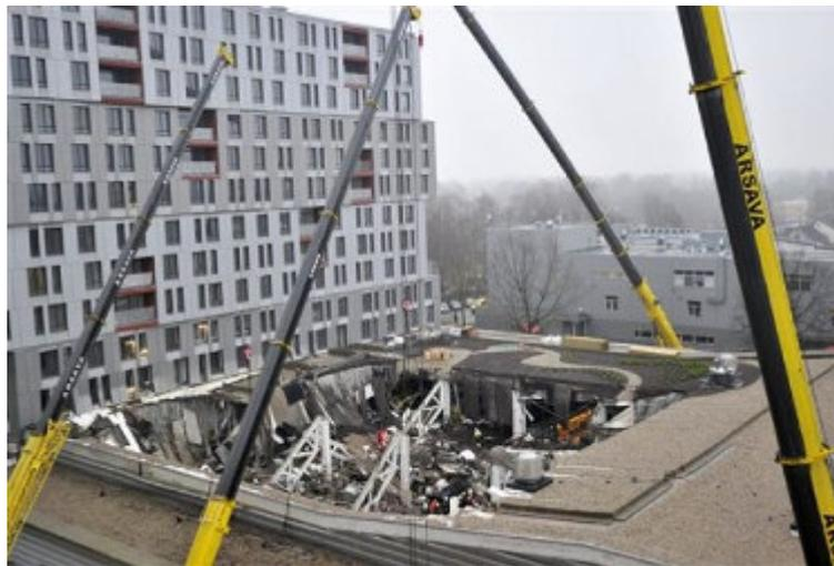
**Fig. 1. Progressive collapse in Riga supermarket Maxima**
