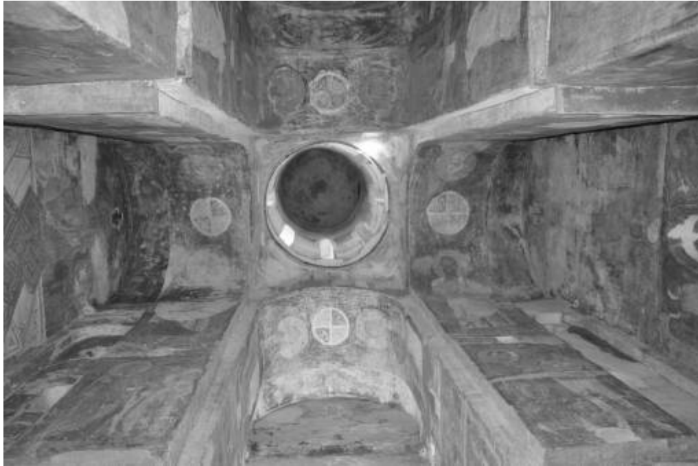
Figure 2 – General view of the church structure. On the walls, arches, pillars, there is a fresco painting of the 12th century
