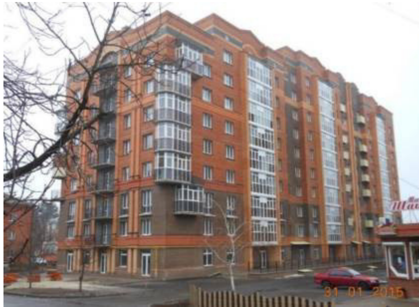
Figure 1 – General view of the three-sectioned nine-ten storey house in the str. V. Kozak, 14 in Poltava (order of sections – left – right)
