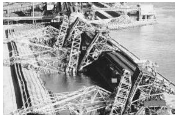
Figure 4 -- Tilting the crane due to the action of seismic forces
