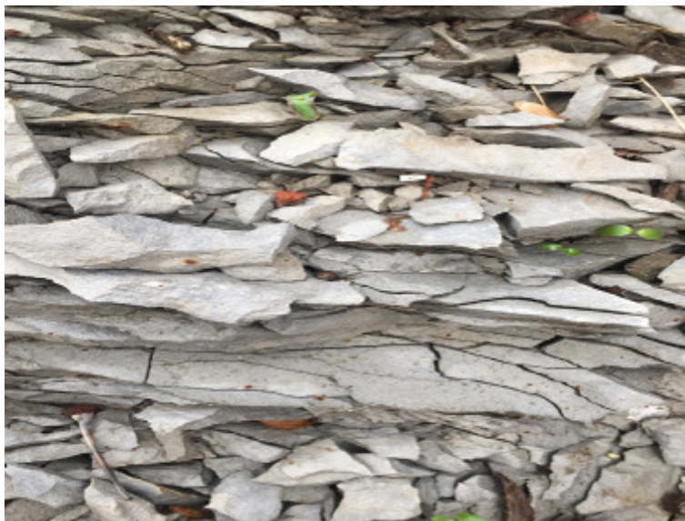
Figure 3 – Material bundle under weather conditions influence
