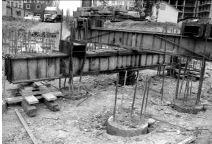
Figure 5 – Fragment of soils testing with bored piles
