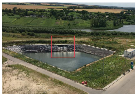
Figure 5 – Soil slope subsidence of south-west side of water basin
