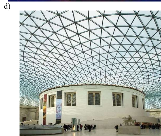
Figure 1 – Examples of the diagrid structural systems:
